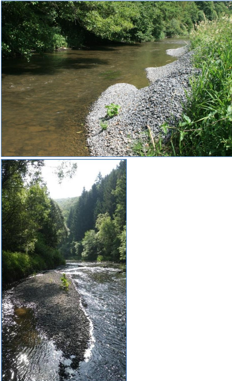
Figure 15: Gravel input and new created gravel banks
