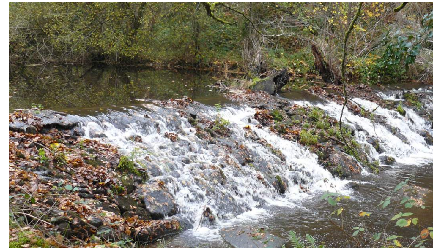
Figure 1 : Dam before restauration
