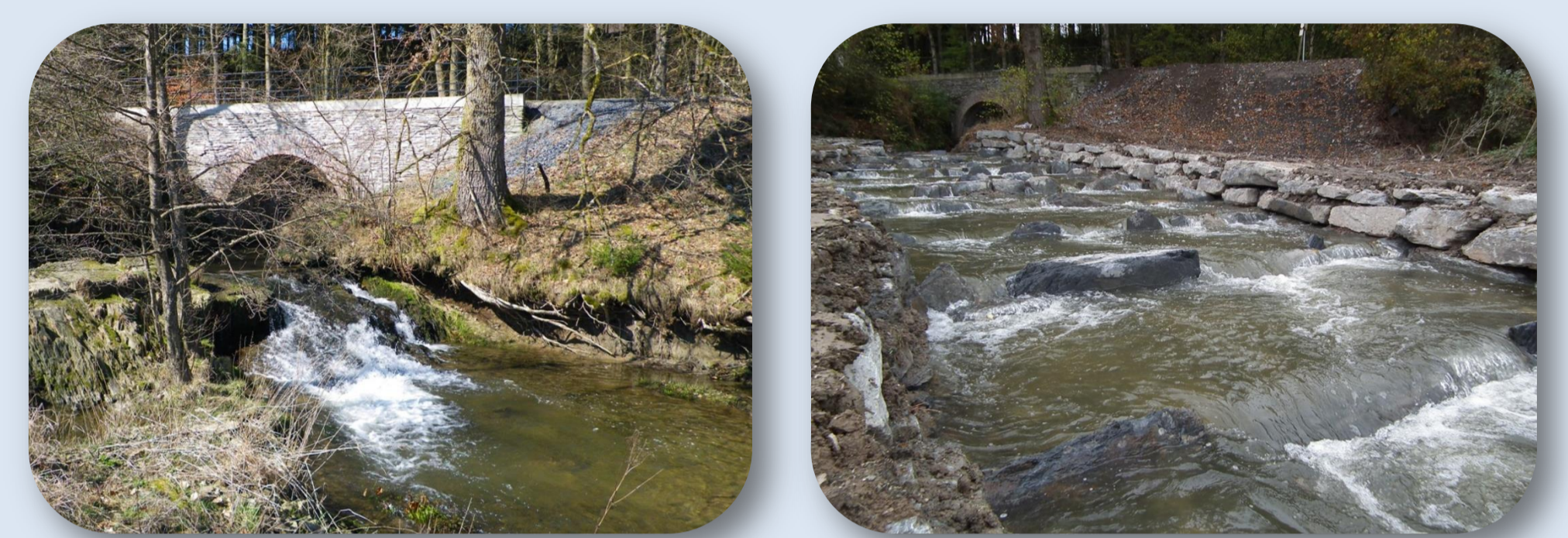
A rock-ramp fishway (5% slope) has been built with 12 transverse ridge rocks forming a series of pools and small falls (0,1 m).
