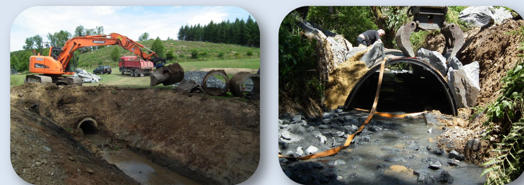
Upstream road crossings have been improved for fish passage and the canalized stream has been uncovered. Downstream barriers were preserved.
