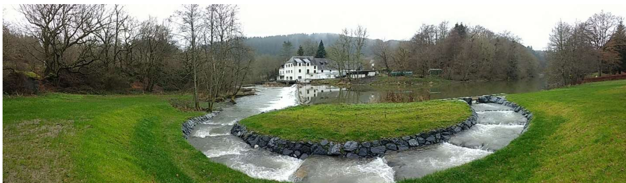
Figure 13: Fish pass in Moulin de Bigonville
