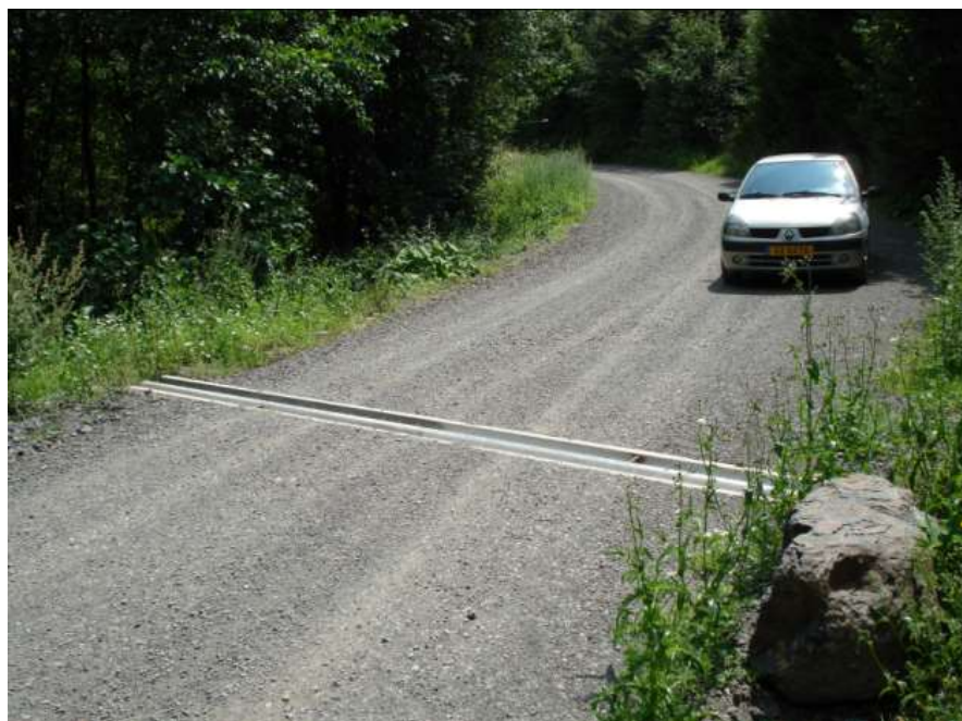
Figure 2: Water evacuation grids at the forest road next to Schwärzerbaach
