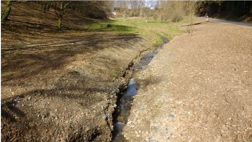
Figure 5: Feierbech – unstable riverbed (February 2017)
